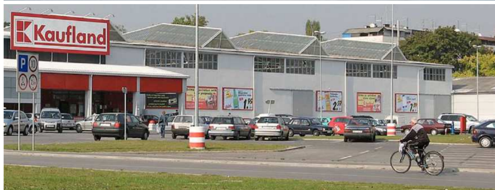
View of a parking lot from which the ongoing promotional event is immediately visible – with six large promotional signs placed on the external wall, using them as a large sales point.
